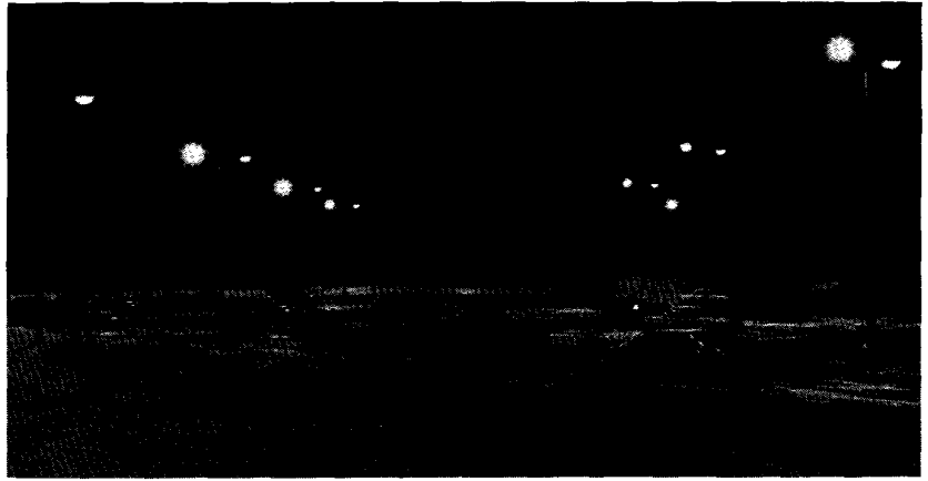
Figure 8. Parking-lot installation of 25 400-watt high-pressure sodium discharge lamps.
