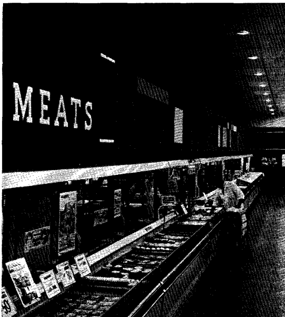
Figure 8. Supermarket meat department in which the major component of illumination is supplied by interference-film lamps. Lamps are medium floods, spaced about eight feet on centers.
