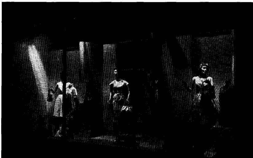
Figure 9. Show window in which general illumination is provided by 500-watt quartz-iodine lamps in wide-beam floodlights and spotlighting is provided by two 300-watt PAR56 interference-film narrow spot lamps aimed at each mannequin.
