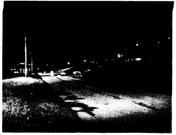
Figure 7. Test installation with open suburban units turned off.
