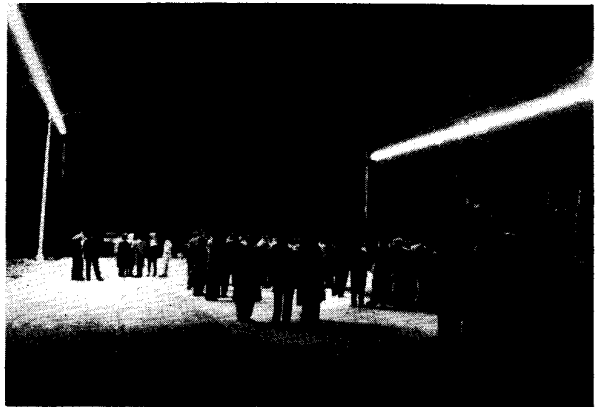
Figure A. Continuous fluorescent strip lighting over a 100-foot section of 70-foot wide roadway. Eight-foot fluorescent floodlighting units equipped with 96T12 cool white rapid start lamps are mounted on catenary 28 feet above the roadway.
