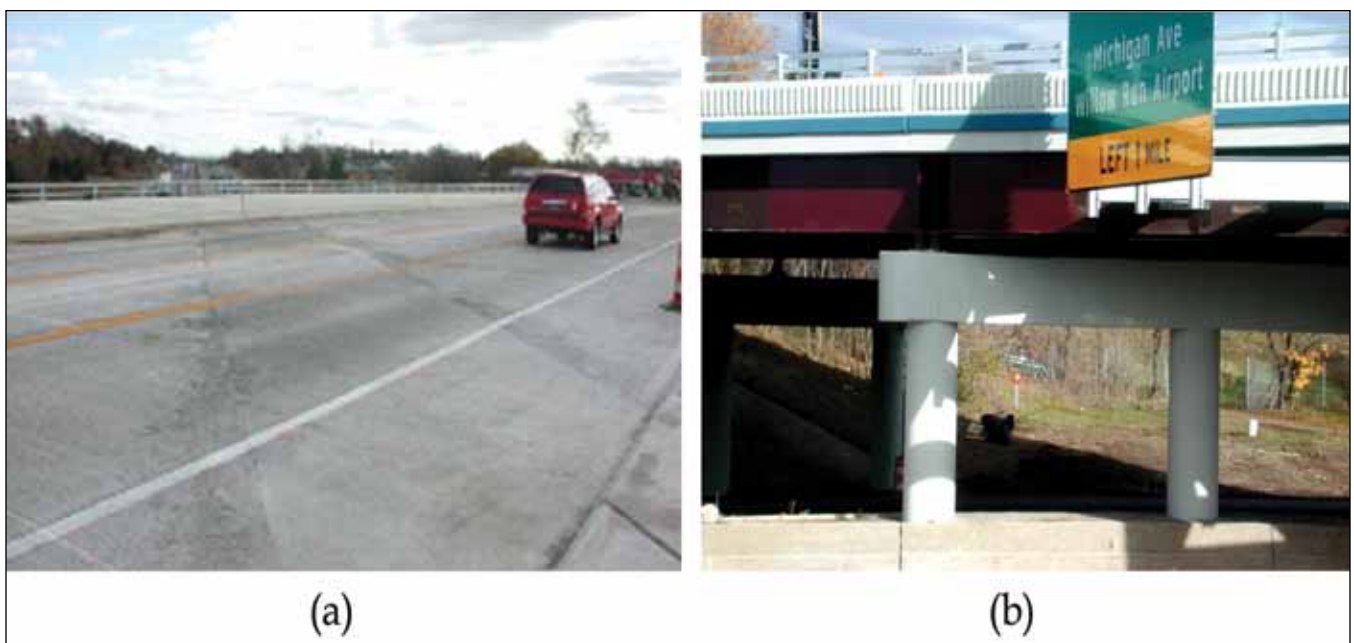
Figure 7. (a) ECC link-slab on (b) Grove Street Bridge in Ypsilanti, MI. Image courtesy of Lepech and Li, 2009.
