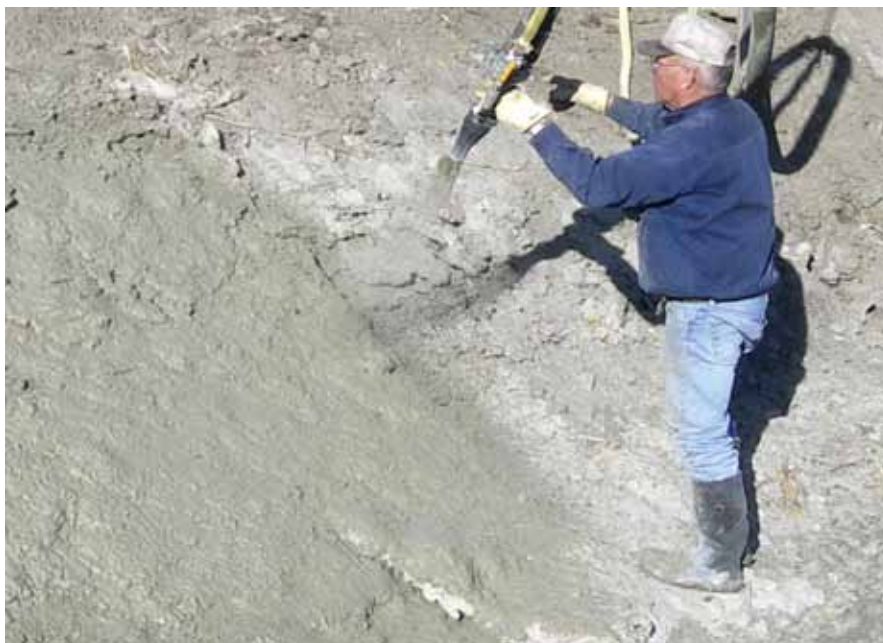
Figure 4. Sprayable ECC applied to irrigation channel repair. Image courtesy of LFL & Associates, 2008.
