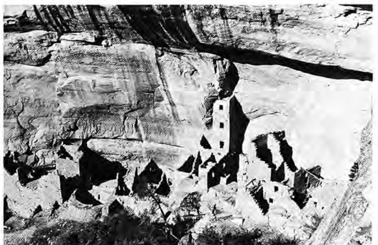
Two views of a highly successful experiment in passive solar design, the elaborate 11th-13th century pueblos of Mesa Verde, Colorado. Warmed with directly gained solar radiation when the sun is at its low winter angle, the stone dwellings are shaded by the overhanging mesatop and cooled by prevailing breezes from the valley below in summer. Heat gain is controlled with massive construction, minimal openings, and stacked space planning.
