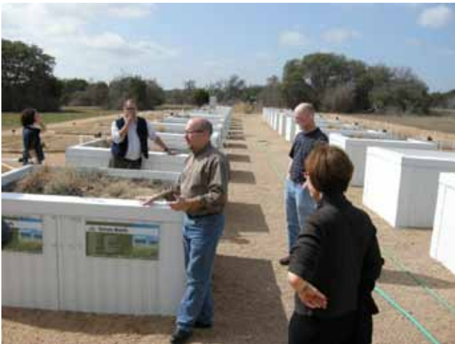
Lady Bird Johnson Center work in progress
