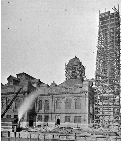
Baltimore, MD sewage lift station.
