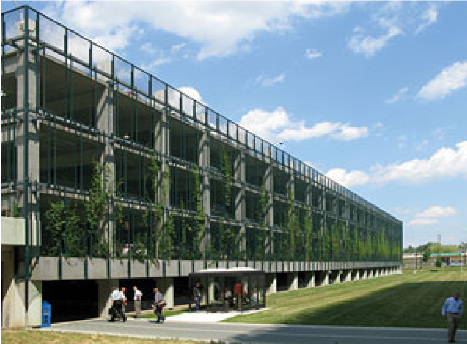
Top left: An example of a simple planted wall on a government parking structure in Maryland. The stainless steel armature can be retrofitted on existing structures along with planting medium and drip irrigation.
